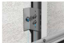
Connection at floor slab and base wall
