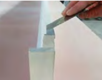
10. When it comes to major repairs, cement sealant should be applied in multiple layers.
