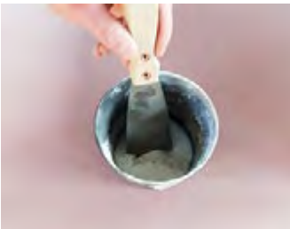
4. Mixing (ratio of liquid adhesive and water 1:10).
