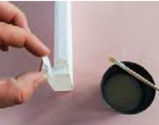
3. After cleaning, the liquid adhesive is applied to the damaged areas.
