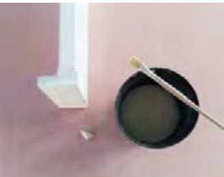
6. First, the surface should be moistened.
