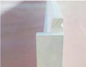
7. Liquid adhesive is applied to the damaged area with a brush or a sponge (in the case that the damaged portion is still part of the panel and the adhesive is pressed into the gap).
